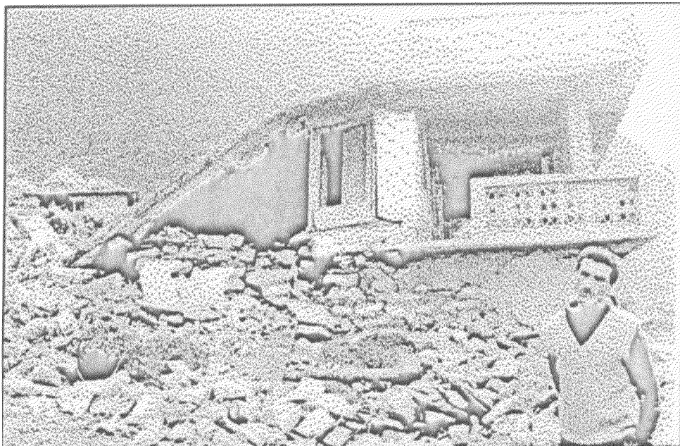
Collapse of RCC slab due to failure of rear wall: Village Ginda, Bhatwari Tahsil, Uttarkashi District
