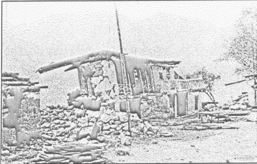
Collapse of building due to failure of masonry wall and settlement of ground storey: Village Maneri, Bhatwari Tahsil, Uttarkashi District
