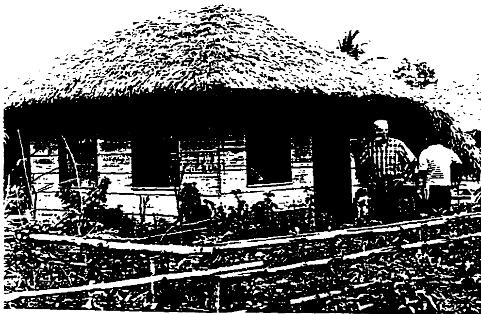
FIGURE 6. NEW DESIGN CORE SHELTER UNIT (CSU) IN USE USING LOCAL MATERIAL ANAHAW ROOFING AND LIGHT TIMBER BOARD SIDING
