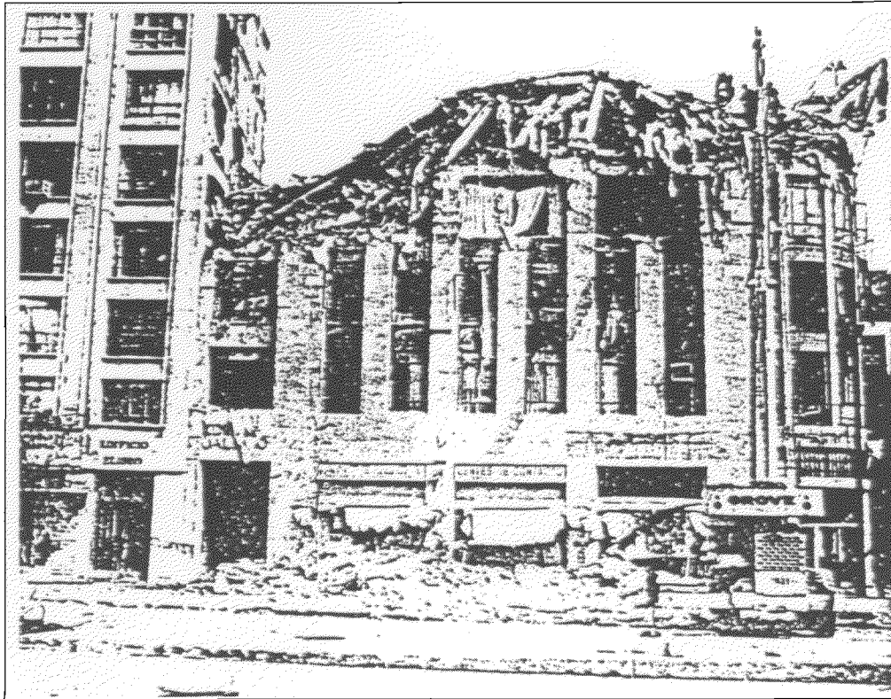
Older concrete building -- upper floor collapse
