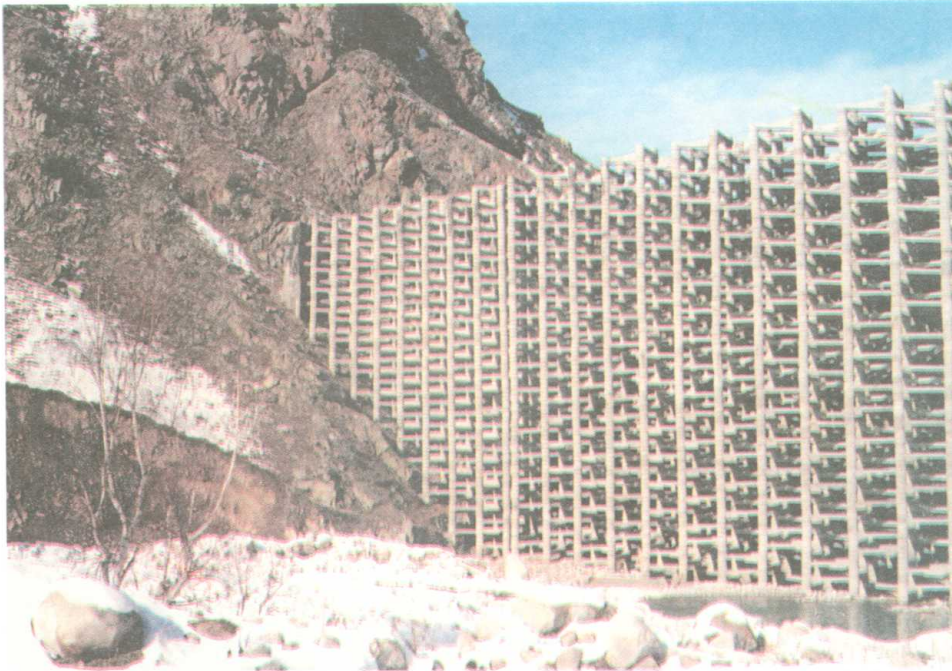
Construction of a mudflow dam.
