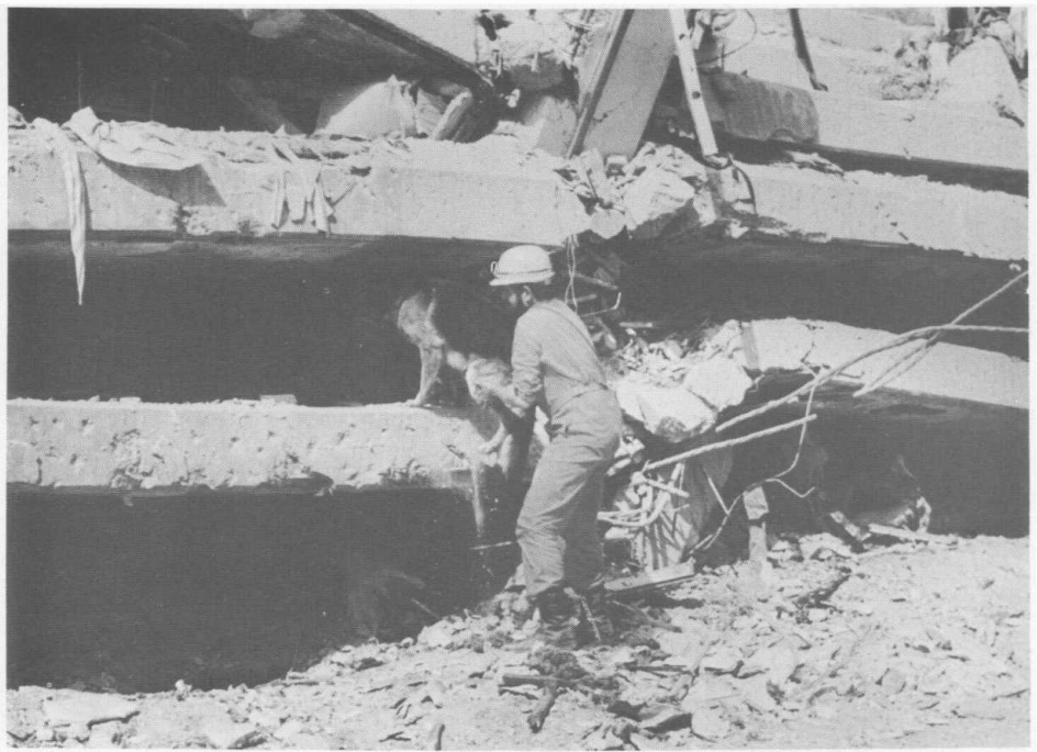
The earthquake released colossal amounts of energy, several storeys were reduced to a height of only 50-80 cms.
