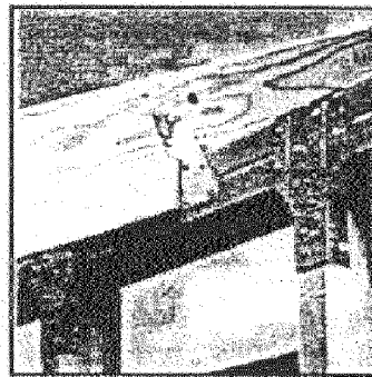
Figure 7. Samples of metal connectors used to secure timber elements.
